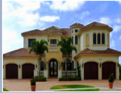
THE OAKS AT BOCA RATON
